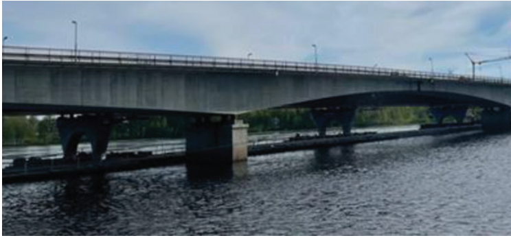
Figure 10. The Kalix Bridge in 2021 (photo courtesy Sas et al. 2024).
