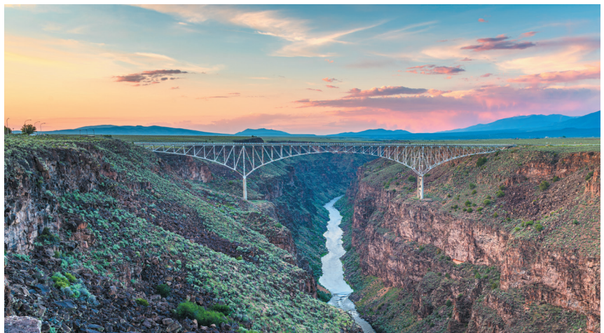
A team of researchers in New Mexico are looking to use fast-developing digital robotic technologies to create a comprehensive robotic-enabled bridge inspection system (pictured: the Rio Grande Bridge in Taos, New Mexico).
