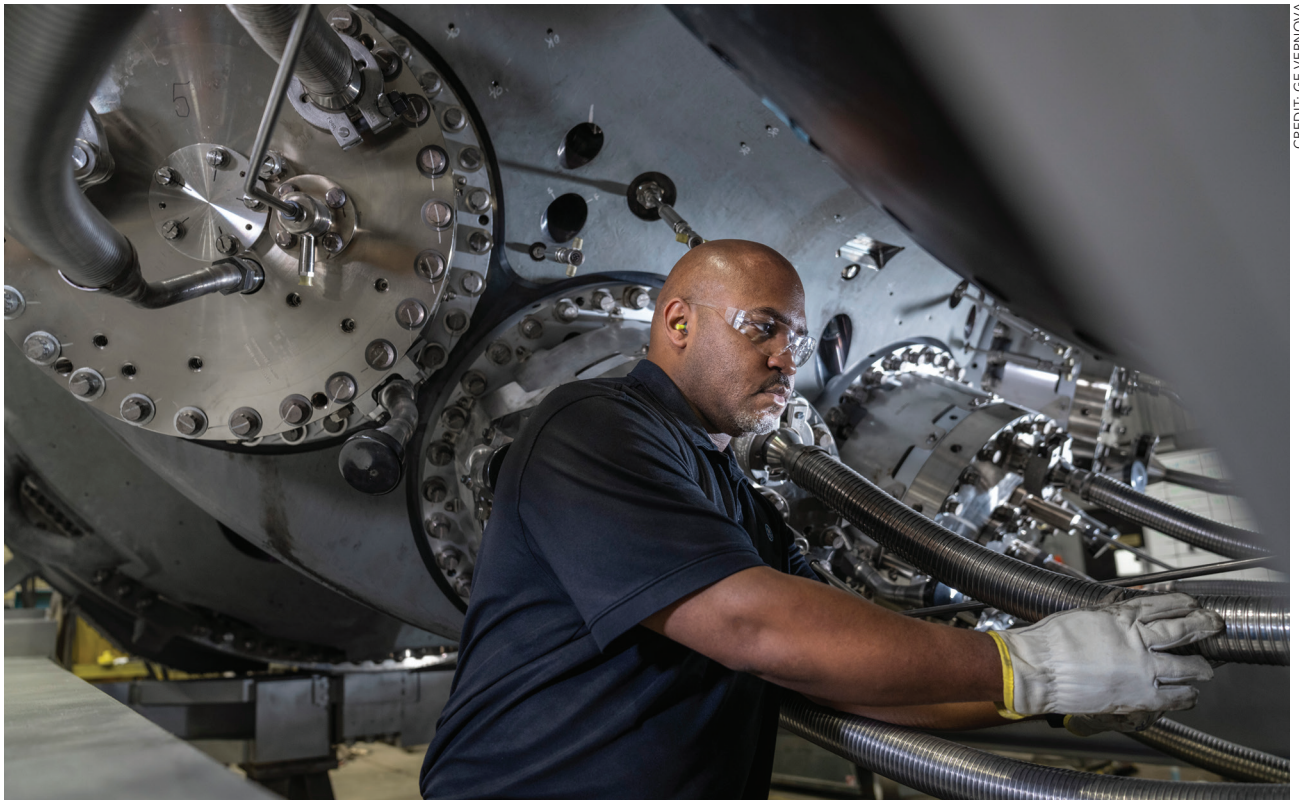
Figure 2. Visual inspection of a GE Vernova large frame gas turbine’s fuel lines.
