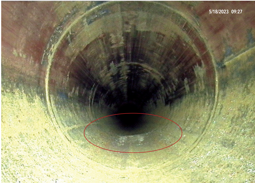
Figure 5. Crawler camera view.
